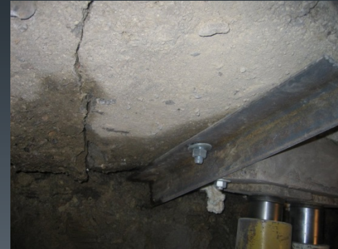
Collapsed Foundation
