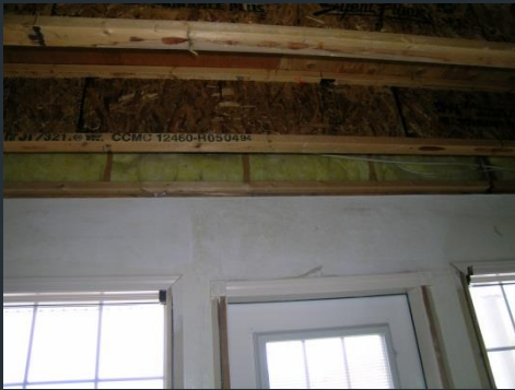
Water Penetration Repair
