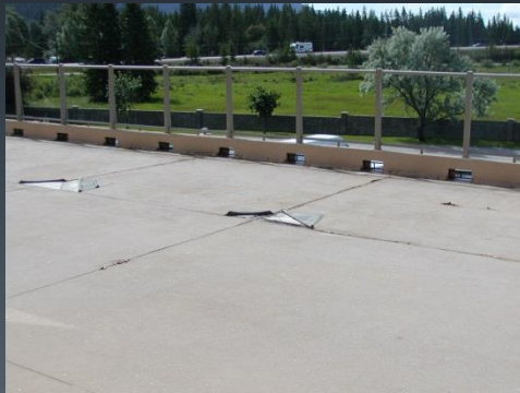
Failed Deck Membrane
