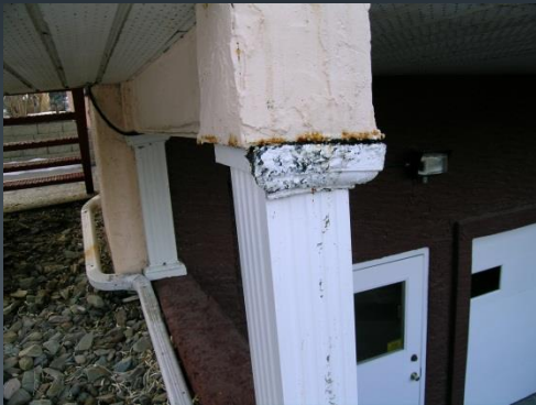
Failed Column & Soffit
