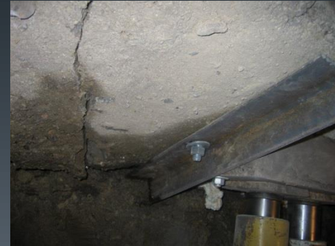
Collapsed Foundation
