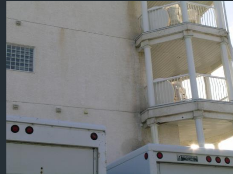
Failed Soffit & Stucco
