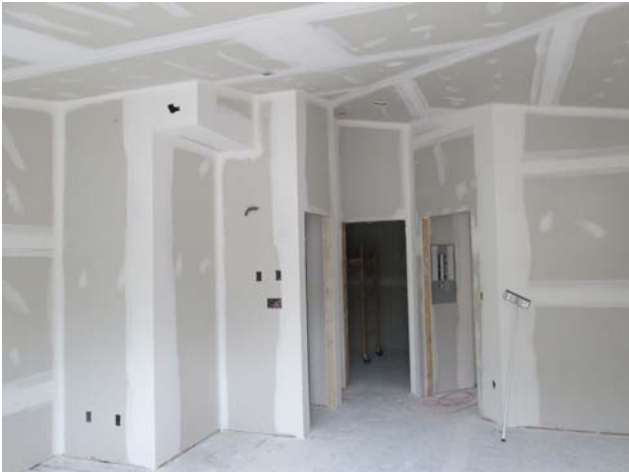
Building 800 – Drywall taping and sanding is generally complete in a further two units.
