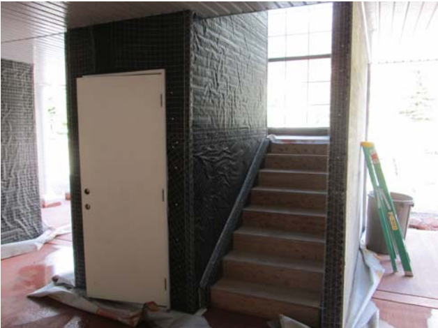
Views of the central stairwell on Building 400. The new stairs have been installed. Walls are ready for stucco.
