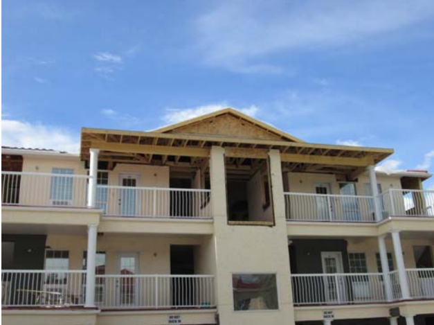
Views of the south (front) elevation of Building 800. Framing of the new roof addition is complete.
