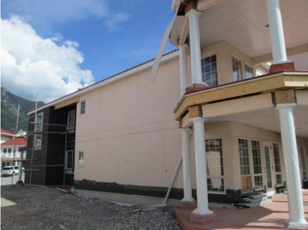
Views of the north elevation of Building 400. Application of the stucco scratch-coat is ready to begin.
