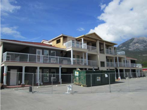
Views of the south (front) elevation of Building 800. Framing of the new roof addition is complete.
