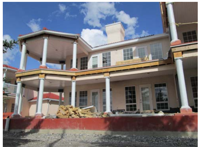
Views of the west (rear) elevation of Building 400. The new columns and soffits have been installed.
