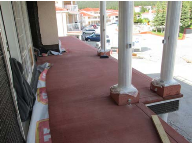
Building 400 – The new concrete topping has been completed on the balconies.
