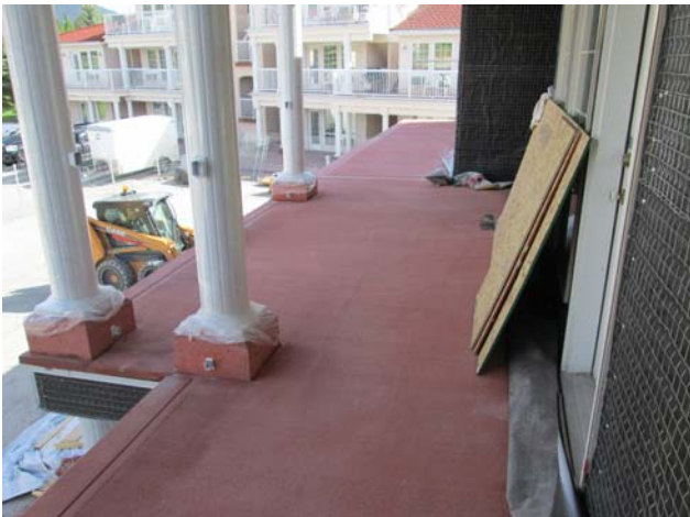
Building 400 – The new concrete topping has been completed on the balconies.
