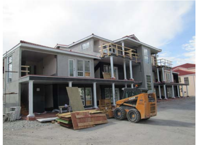
Views of the east (front) elevation of Building 400. Stucco replacement work is well advanced.
