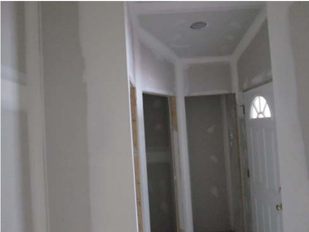
Building 800 – Drywall taping and sanding is generally complete in a further two units.
