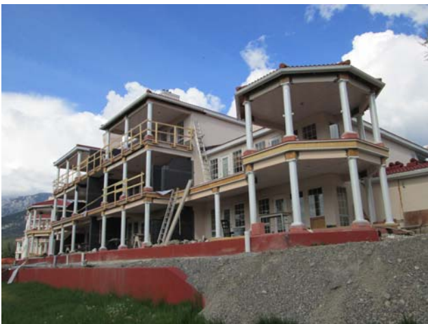
Views of the west (rear) elevation of Building 400. The new columns and soffits have been installed.
