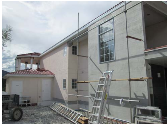
Views of the south elevation of Building 400. The new stucco scratch-coat is generally complete.
