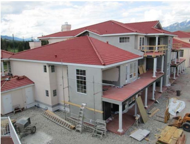
Views of the south elevation of Building 400. The new stucco scratch-coat is generally complete.
