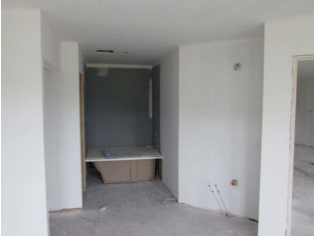
Building 800 – Prime painting is generally complete in two of the units.
