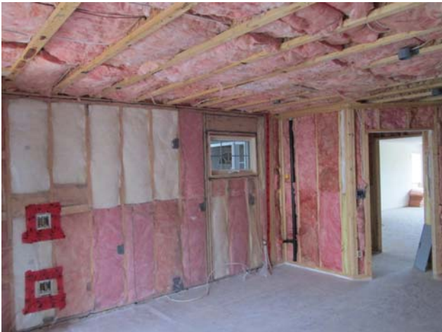
Building 800 – Drywall boarding remains to be completed in four of the ten units.
