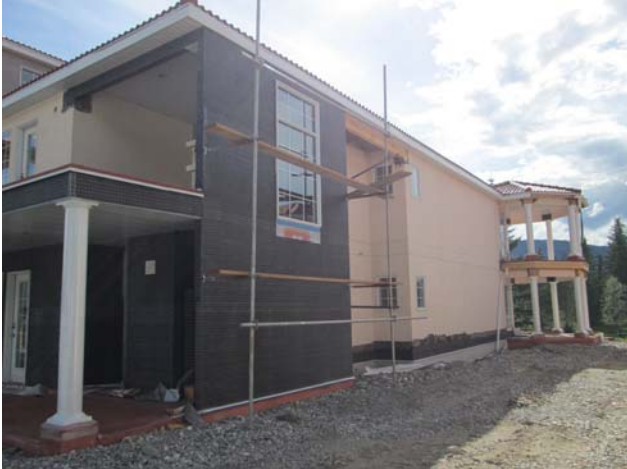
Views of the north elevation of Building 400. Application of the stucco scratch-coat is ready to begin.
