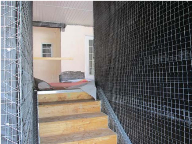
Views of the central stairwell on Building 400. The new stairs have been installed. Walls are ready for stucco.
