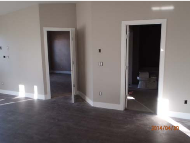
Further view of the finishing in building 300.
