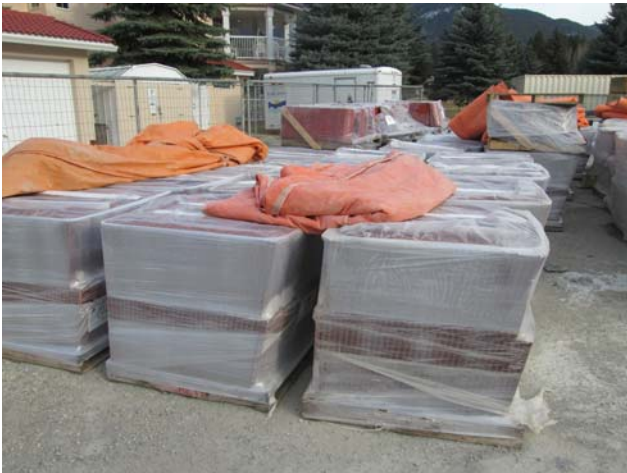
The roof tiles for building 300 are on site.
