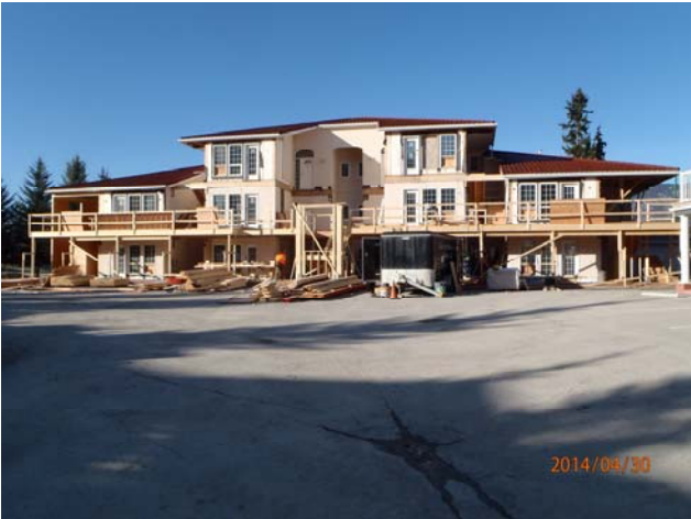
View of the north (front) elevation of building 300.
