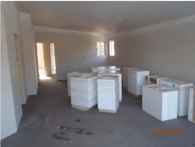
View of the cabinets delivered for building 400.
