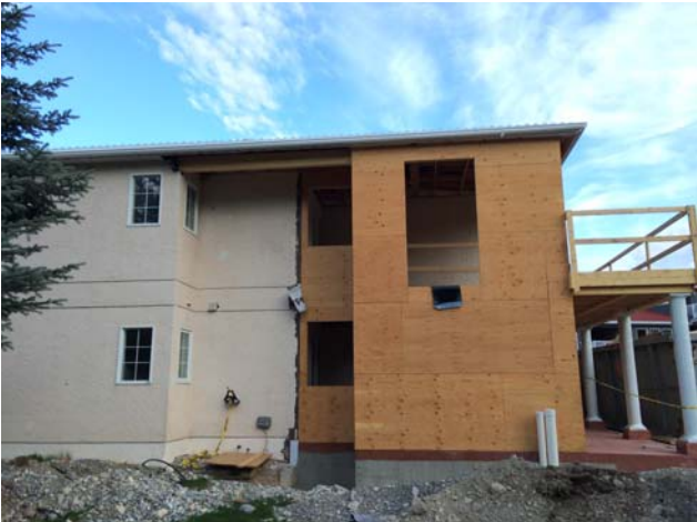
View of the east and west elevation of building 300. The corner stairwells have now been framed.
