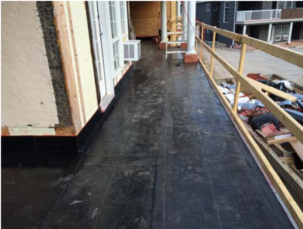
Building 300 – Installation of the waterproof membrane is well advanced on the upper balconies (north side).
