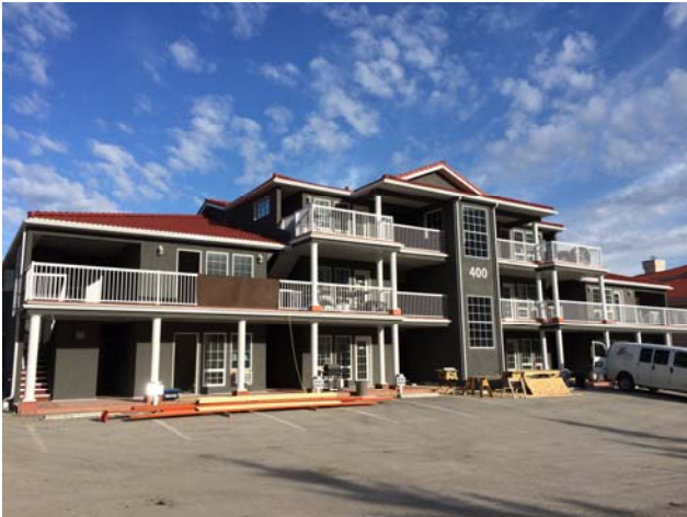
View of the east (front) elevation of building 400.
