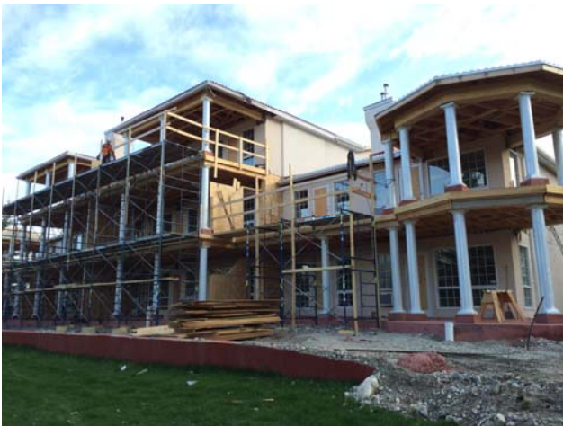
Views of the south elevation of building 300. Balcony and roof framing is complete.
