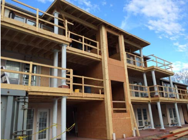
Framing of the new central stairwell is complete.
