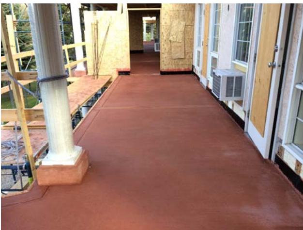
Building 300 – The concrete floor topping has now been poured on the south side balconies.
