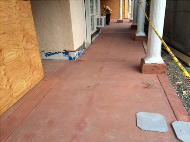
Building 300 – The new suspended concrete patio has been completed along the north (front) side.
