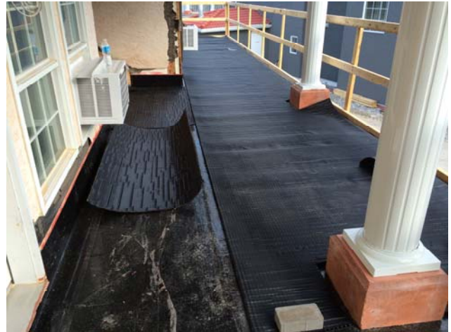
Building 300 – Installation of the waterproof membrane is well advanced on the upper balconies (north side).
