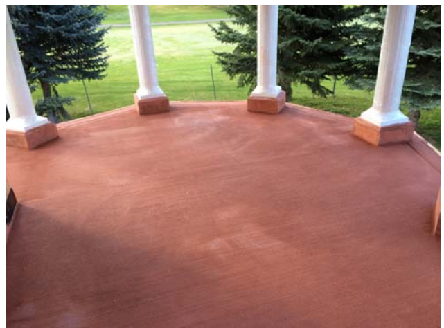
Building 300 – The concrete floor topping has now been poured on the south side balconies.
