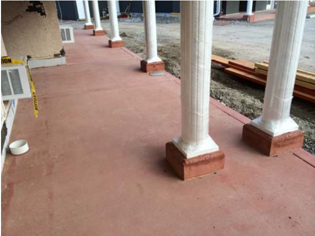
Building 300 – The new suspended concrete patio has been completed along the north (front) side.
