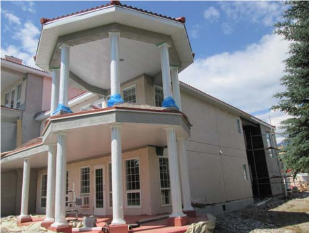
View of the rear balcony at the southeast corner.
