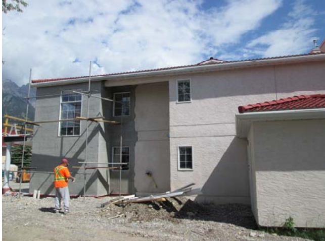
View of the west elevation of building 300.
