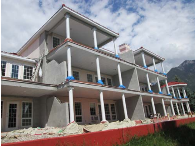
View of the south elevation of building 300.
