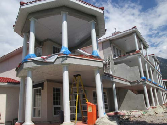
View of building 300 at the southwest corner.
