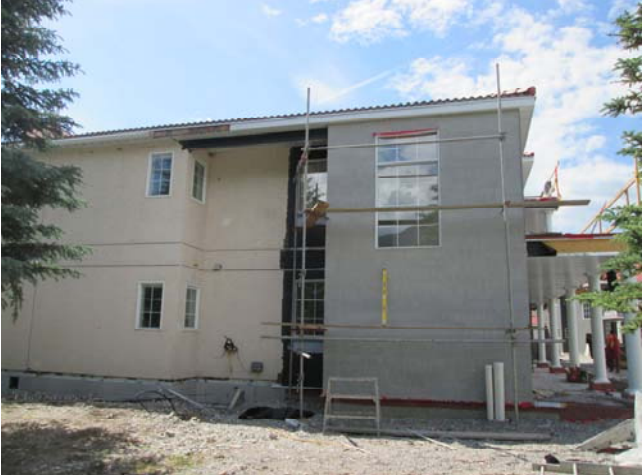
View of the east elevation of building 300.
