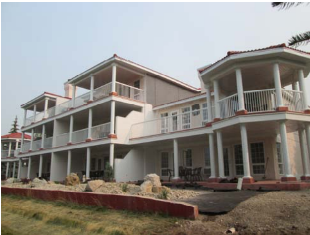
The guardrails have been installed along the south elevation, and the patio furniture has been delivered.
