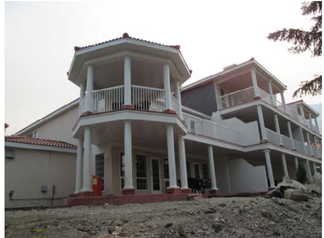
View of the south elevation at the S.W. corner.
