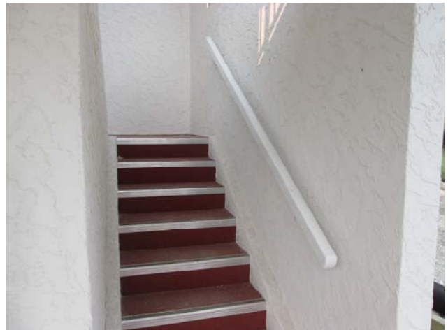
Building 300 – Patching of the stucco is now complete. The stair handrails have been installed.
