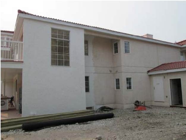
View of the west elevation of building 300.
