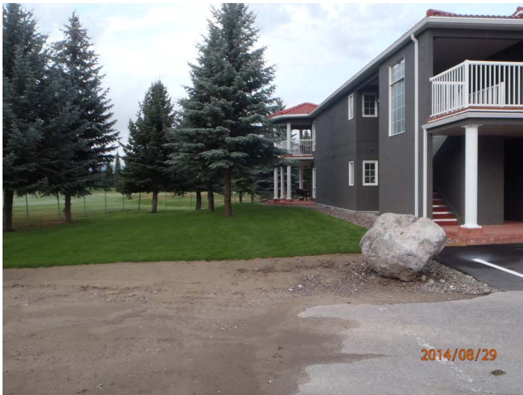
View of the east elevation of building 300, and the landscaping on the east side.
