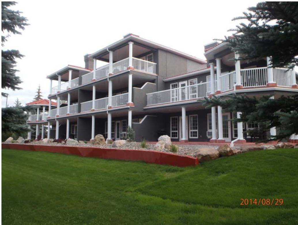
View of the south elevation of building 300.
