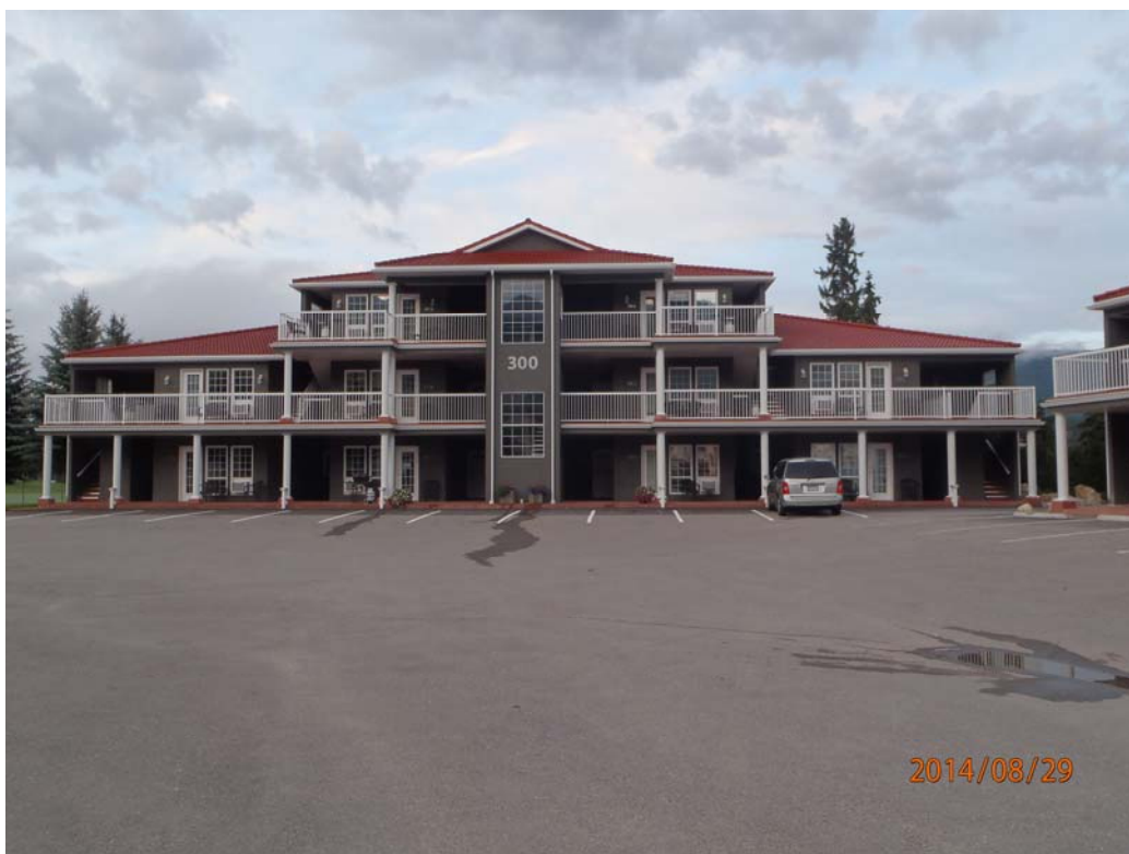
Views of the north (front) elevation of building 300.
