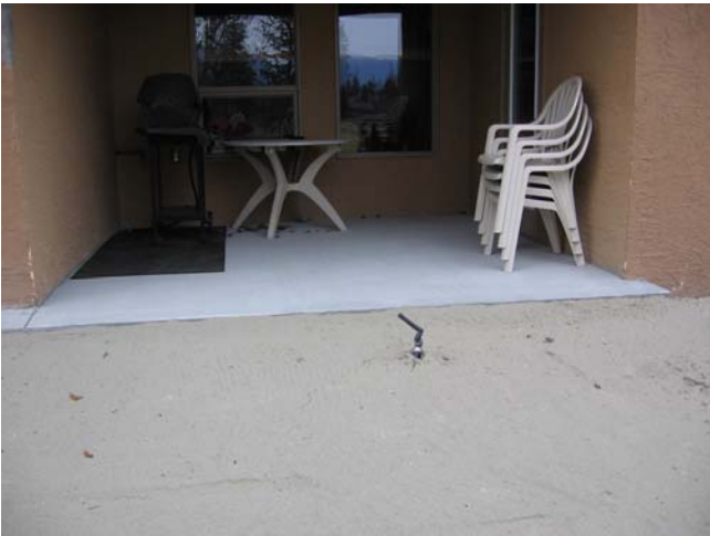
11. New Concrete Slabs-on-Grade to Rear Patios
