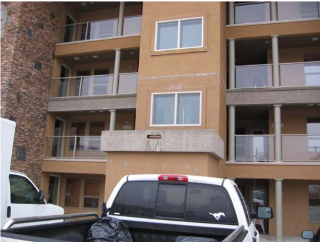
1. Front Elevation Showing Canopy Removed & Stucco Repairs
