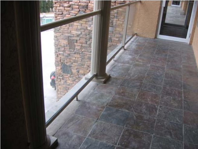
6. 3 rd Floor Balcony Edge Repairs
