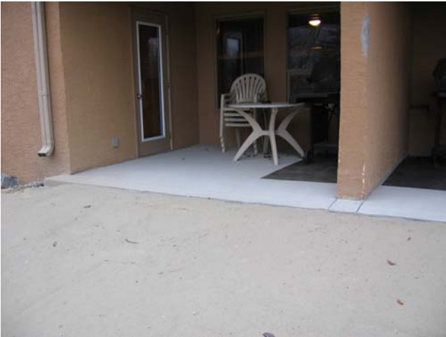
9. New Concrete Slabs-on-Grade to Rear Patios
