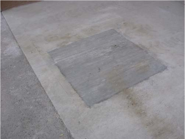
8. Concrete Patching Where Column Removed
