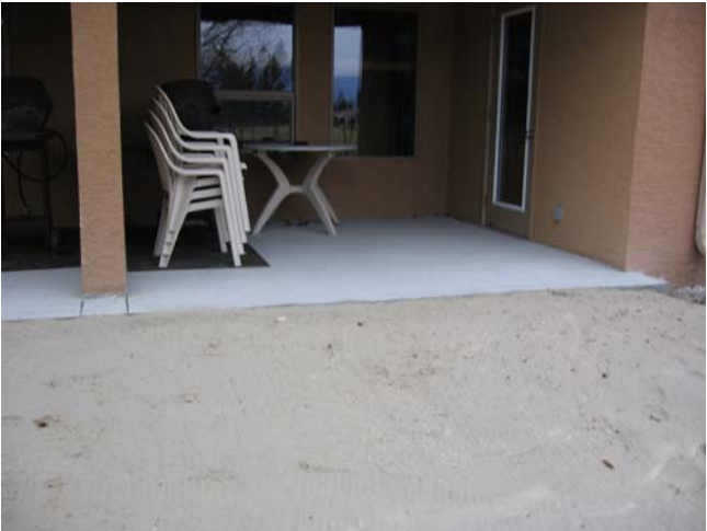
10. New Concrete Slabs-on-Grade to Rear Patios
