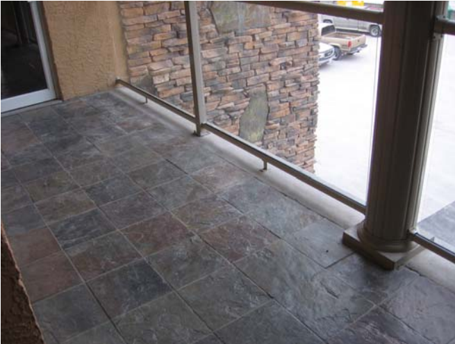
5. 3 rd Floor Balcony Edge Repairs
