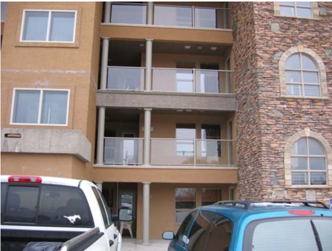
2. Front Elevation Showing Canopy Removed & Stucco Repairs
