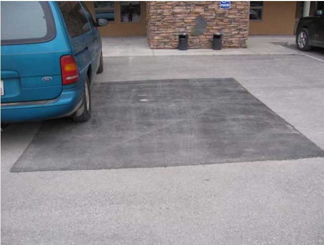
3. Asphalt Patching Where Columns Removed
