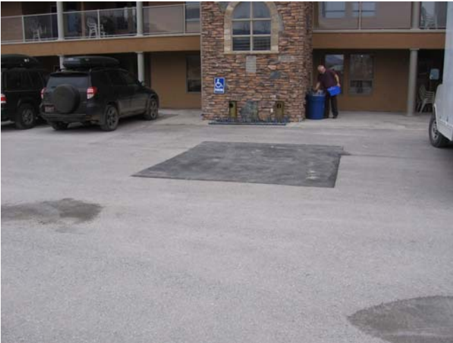
4. Asphalt Patching Where Columns Removed
