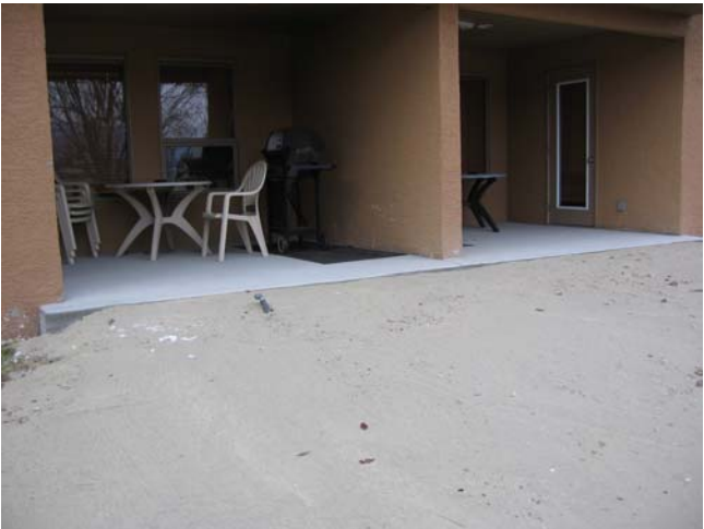
12. New Concrete Slabs-on-Grade to Rear Patios
