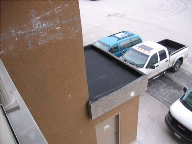
7. Elevator Machine Room Roof
