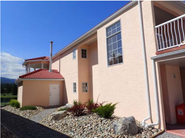
View of the west elevation of building 500.
