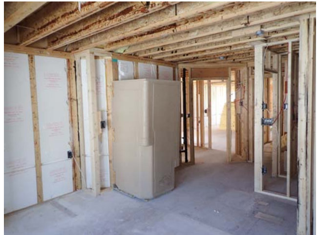
Building 500 – Views of the living area in Unit 201B. Demolition work is complete. New partitions framed.
