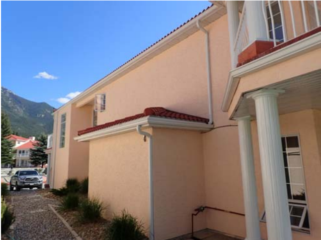
View of the east elevation of building 500.
