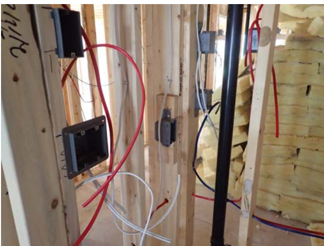
Building 500 – Views of the electrical and plumbing rough-in work underway in Unit 201A.
