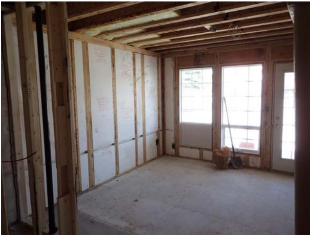
Building 500 – Views of the living area in Unit 201B. Demolition work is complete. New partitions framed.
