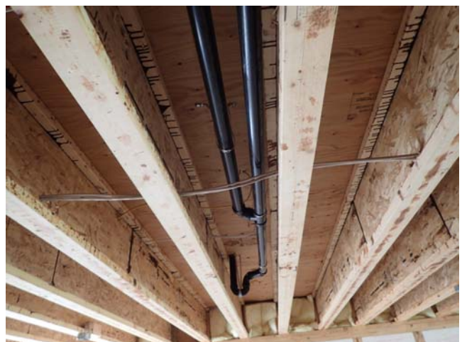
Building 500 – Views of the electrical and plumbing rough-in work underway in Unit 201A.
