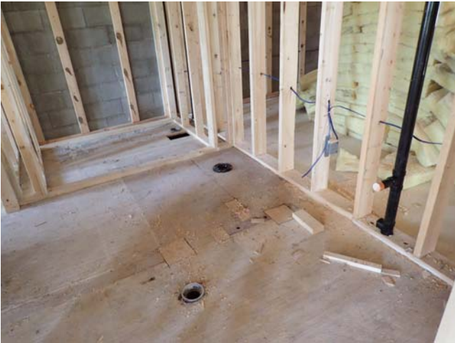
Building 500 – Views of the bathroom in Unit 201A. New partition framing is complete. New tub delivered.
