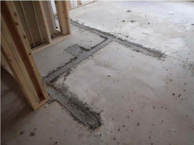
Building 500 – Views of the concrete floor patching completed in Unit 506A and B.
