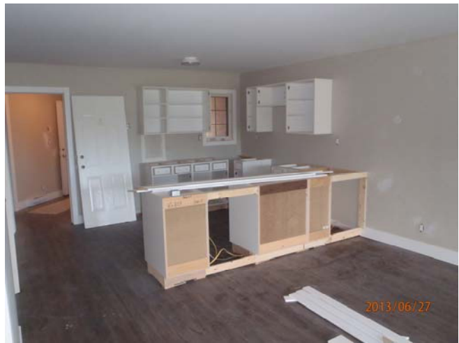
Building 800 – Views of the 'A' unit show suite. Finishing work is nearly complete. Cabinets are installed.
