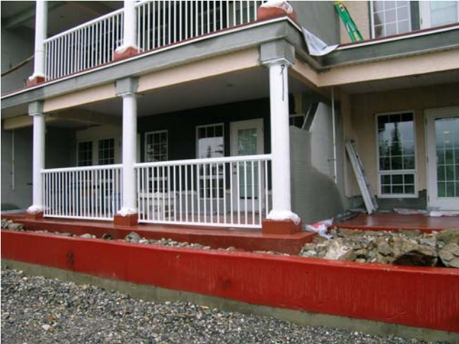
Building 400 – Installation of balcony guardrails and application of the stucco is nearly complete.
