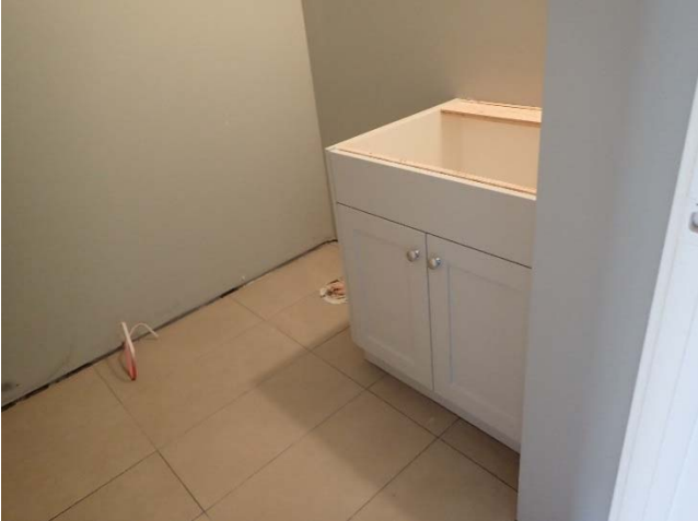
Building 500 – Views of a ‘B’ unit bathroom. The vanity cabinet has been installed, and the tile has been placed.
