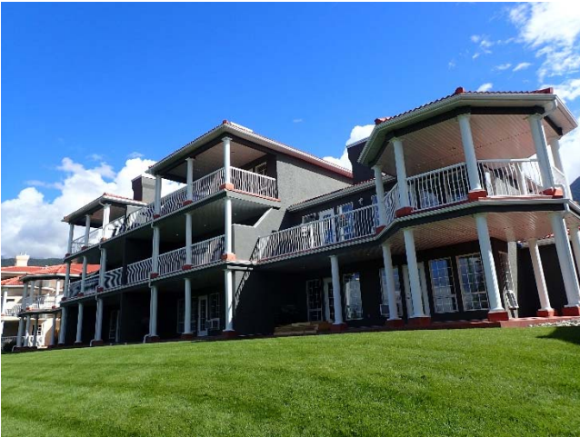
View of the north elevation of building 500.
