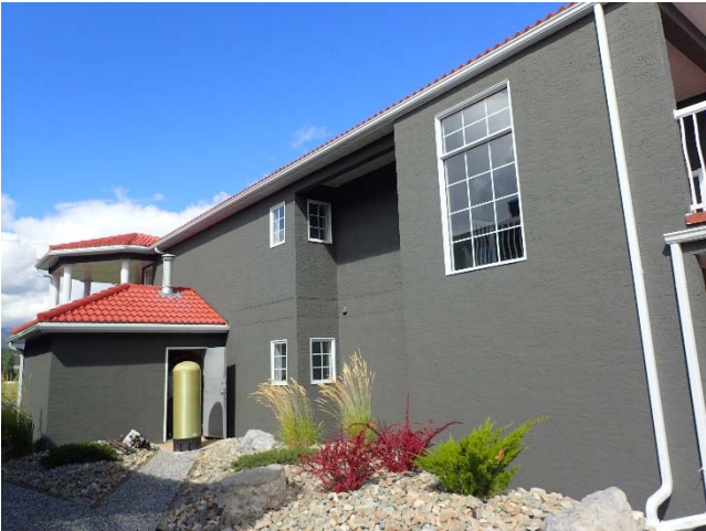
View of the west elevation of building 500.
