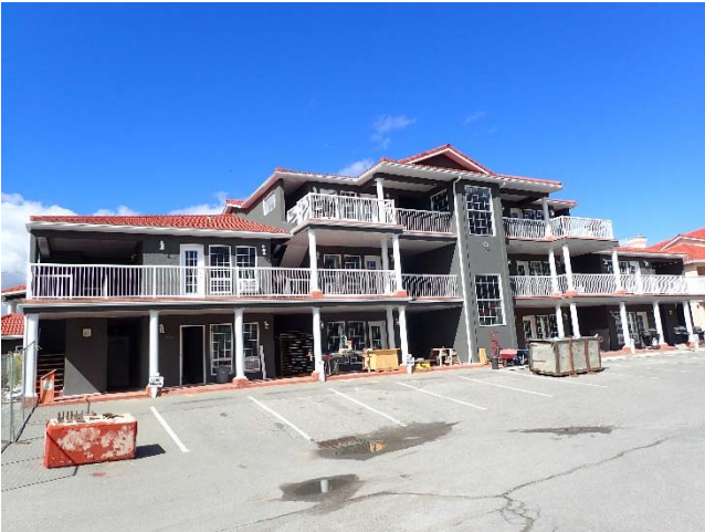
View of the south (front) elevation of building 500.
