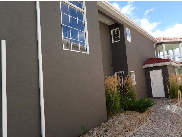
View of the east elevation of building 500.
