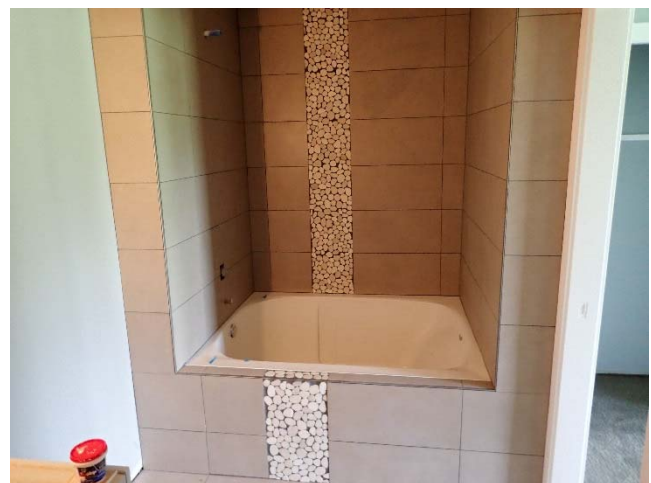
Building 500 – Views of a bathroom in a main floor ‘A’ unit. The tile has been placed, and grouting is underway.
