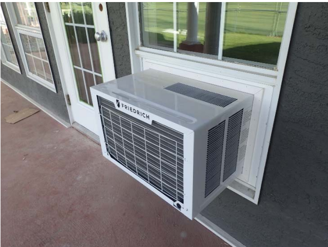
The new air conditioning units have now been installed.
