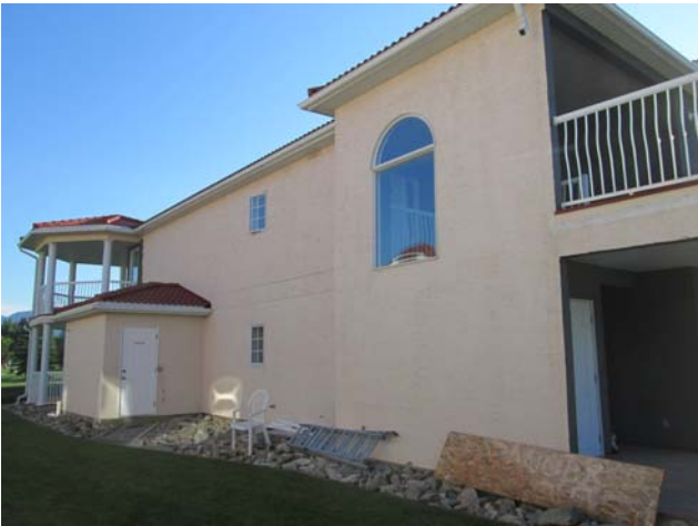
View of the west (side) elevation of Building 800.
