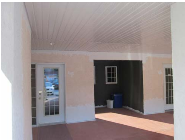
Building 400 – Painting of the stucco is well underway.
