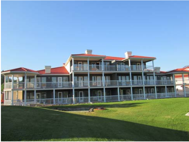
View of the north (rear) elevation of Building 800.
