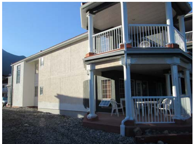
Building 400 – Views of the west elevation and north elevation. Stucco repairs are now complete.
