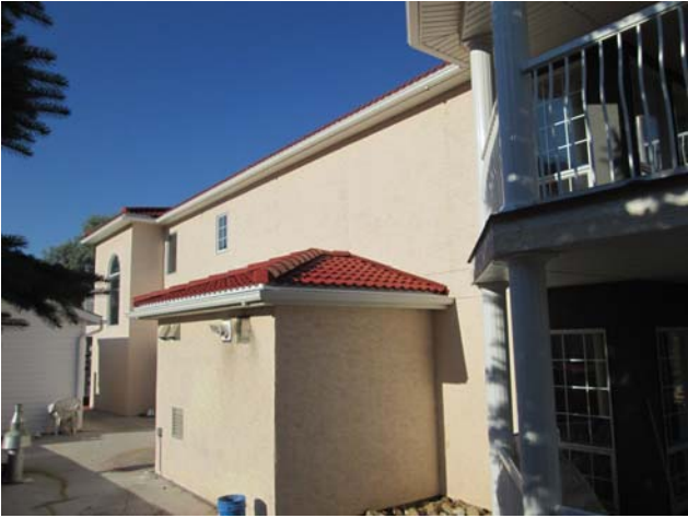
View of the east (side) elevation of Building 800.
