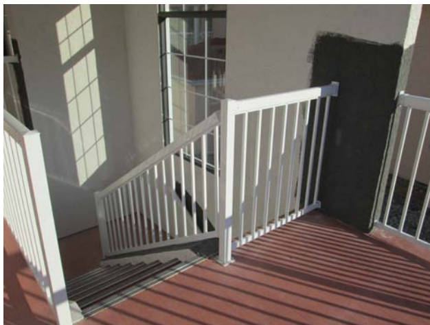
Building 400 – Further views of the guardrails and stucco repairs at the second floor.
