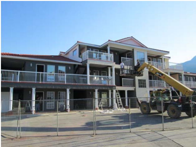
View of the south (front) elevation of Building 800.
