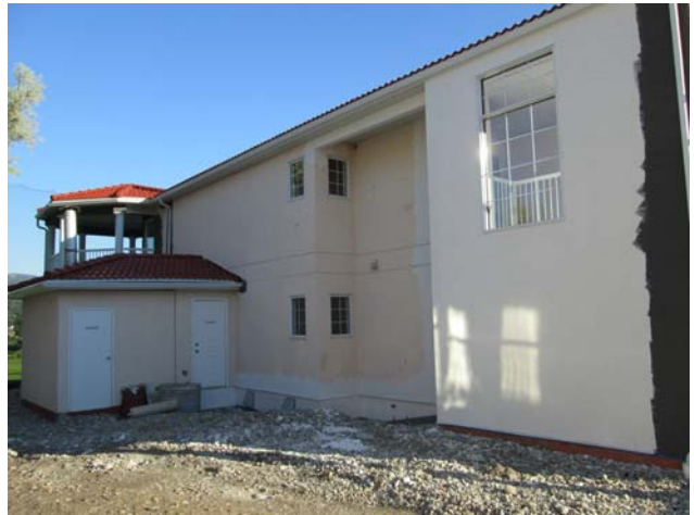
View of the south (side) elevation of Building 400.
