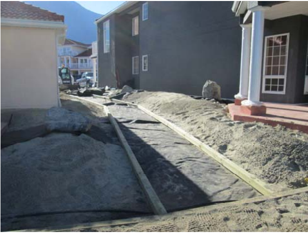
Formation of the stone walkway is well advanced.
