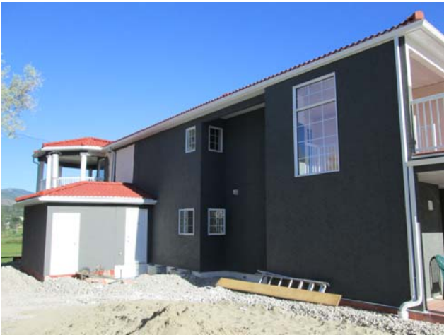
View of the south elevation of Building 400.
