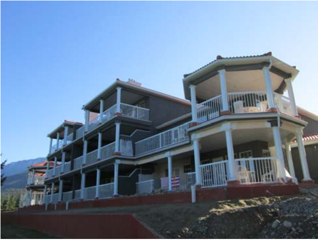
View of the west (rear) elevation of Building 400.
