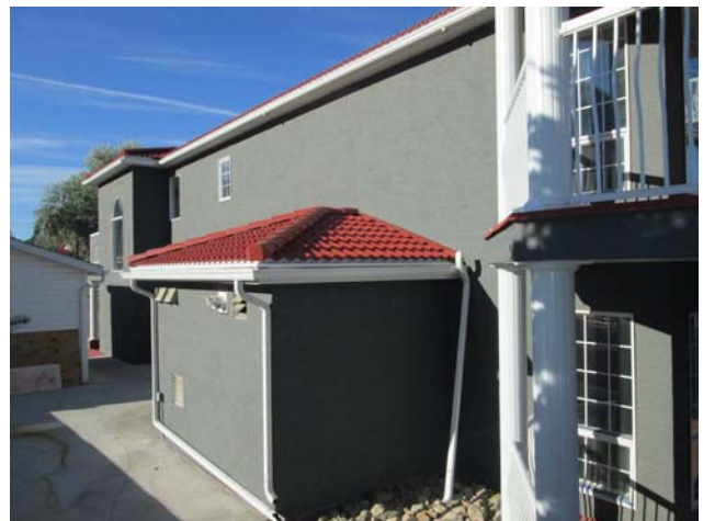
View of the east elevation of Building 800.
