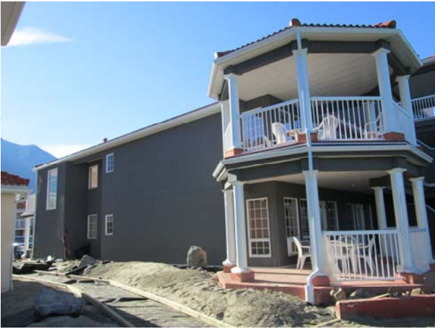
View of the north elevation of Building 400.
