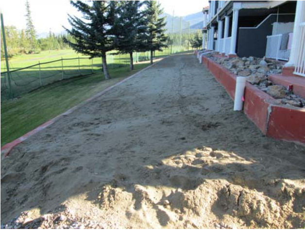
Landscaping remediation is underway.
