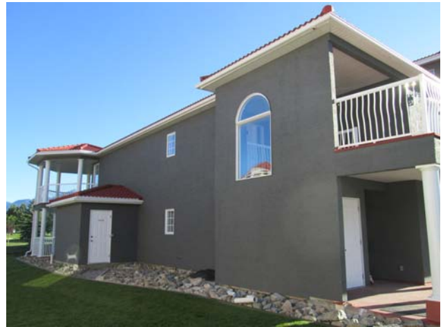
View of the west elevation of Building 800.
