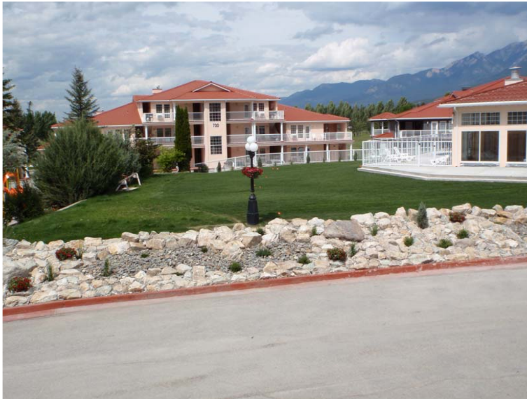
Soft landscaping work has now been completed.
