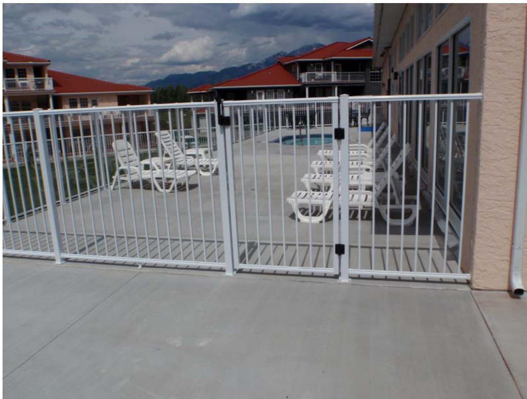
View of the new patio area. The guardrails and gate have been installed. The whirlpool is operational.
