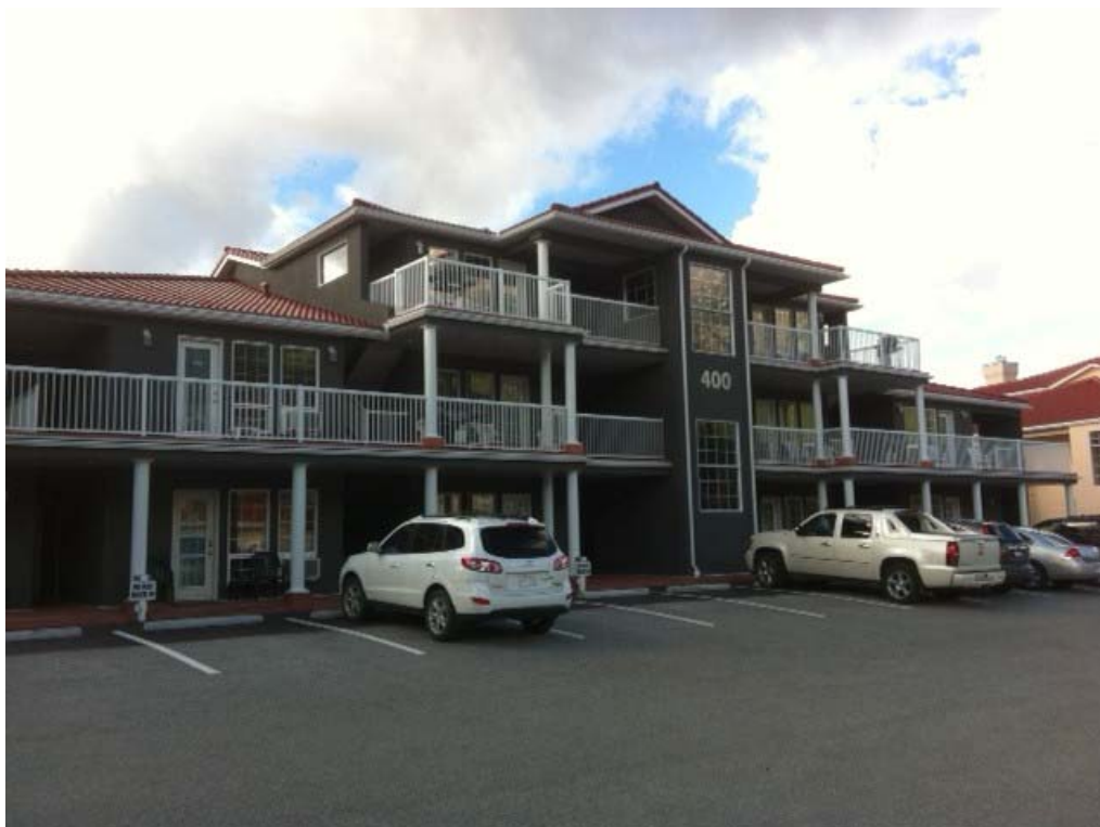
Painting of the exterior stucco has now been completed.
