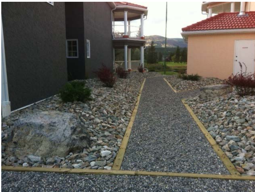
The gravel pathway and surrounding landscaping have been completed between Building 400 and 500.
