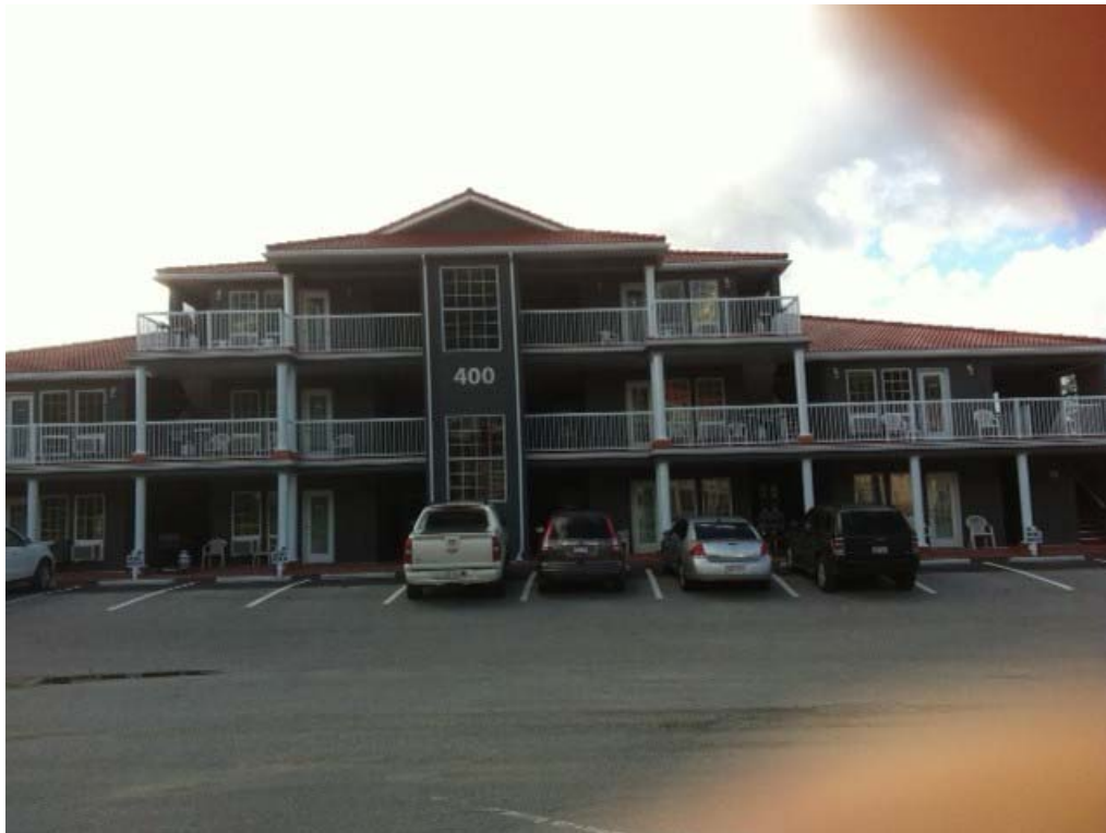
View of the east (front) elevation of Building 400. The new number signage has been installed.
