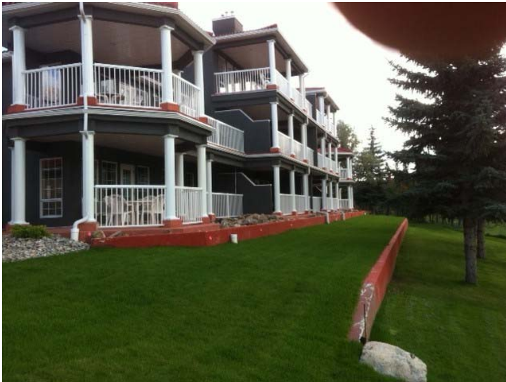
View of the west (rear) elevation of Building 400. Painting is complete. The new sod has been placed.
