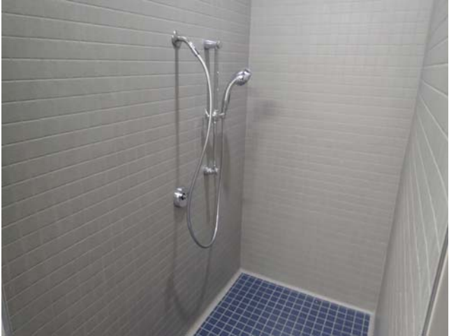
Views of the women's change room showers. Tile work is complete and the fixtures have been installed.
