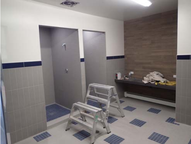
Views of the women's change room showers. Tile work is complete and the fixtures have been installed.
