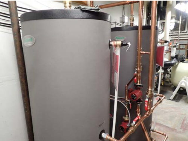
View of the new boilers and hot water tanks installed in the mechanical room.
