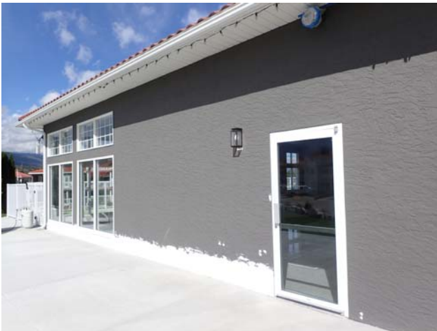
Patching of the stucco has now been completed. Painting of the stucco is nearly complete.
