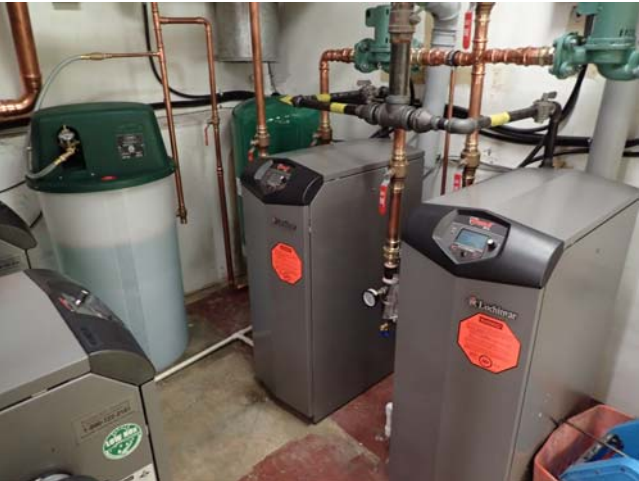
View of the new boilers and hot water tanks installed in the mechanical room.
