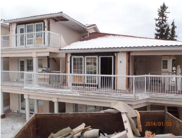
Views of the north (front) elevation of Building 300. Removal of the existing stucco is well underway.
