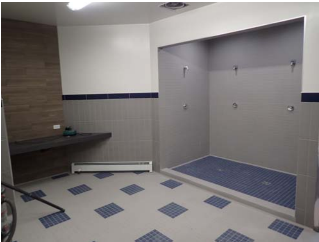
Views of the men's washroom and change room. Tile work is complete and the counters have been installed.
