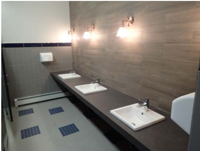
Views of the women's washroom. The tile, vanity, toilet partitions, and fixtures have been installed.
