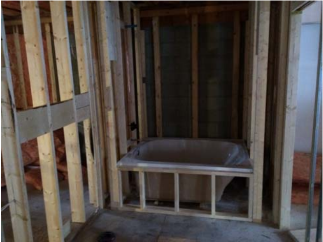
Building 300 – The prefab shower stalls and tubs have been installed. Rough-in work is generally complete.
