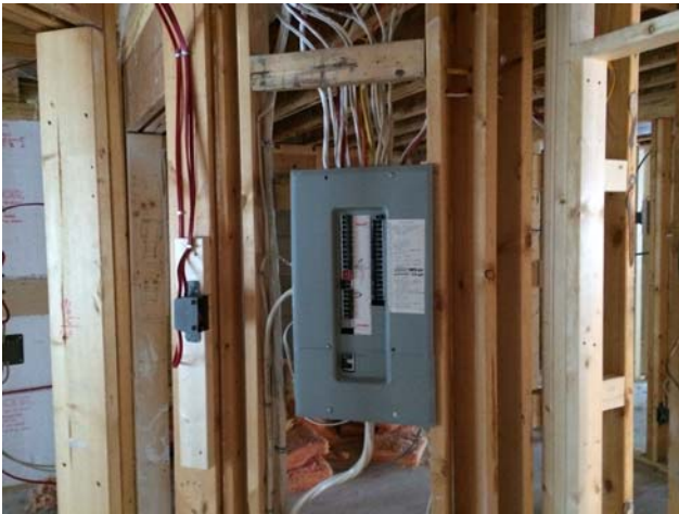
Building 400 – Further views of the new electrical rough-in work that has been completed.
