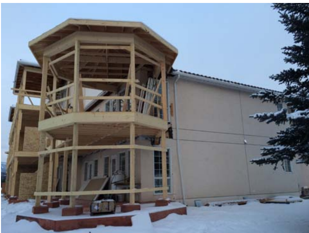
Views of the east and south elevation of Building 300. Framing of the new balconies is now complete.
