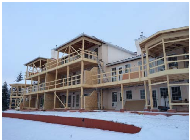
Views of the east and south elevation of Building 300. Framing of the new balconies is now complete.
