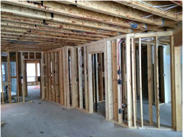
Building 400 – Interior demolition work remains ongoing. New framing has been completed in several units.
