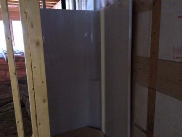
Building 300 – The prefab shower stalls and tubs have been installed. Rough-in work is generally complete.
