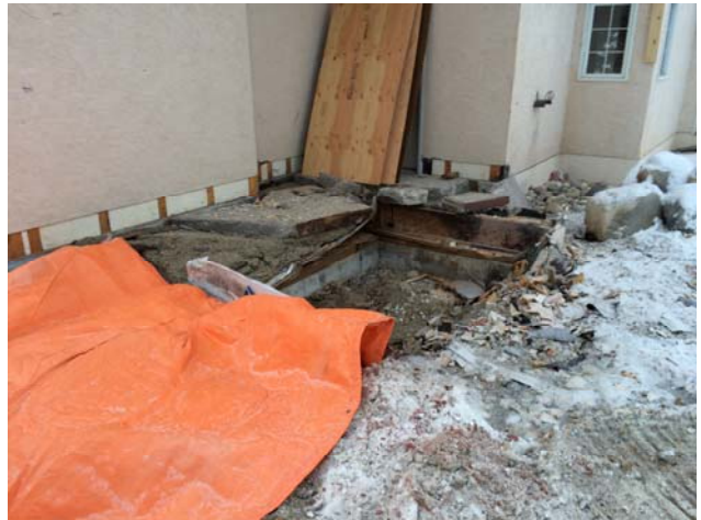
View of the N.W. exterior stairwell foundations.
