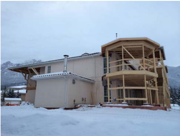
View of the west elevation of Building 300.
