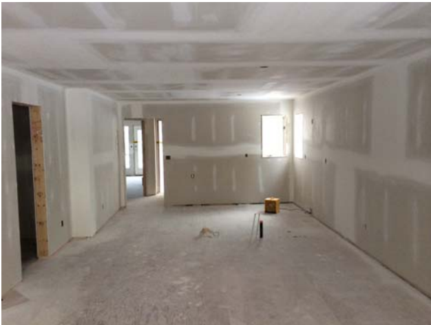
Building 300 – Views of a ground floor unit on the east side of the building. The new drywall is paint ready.
