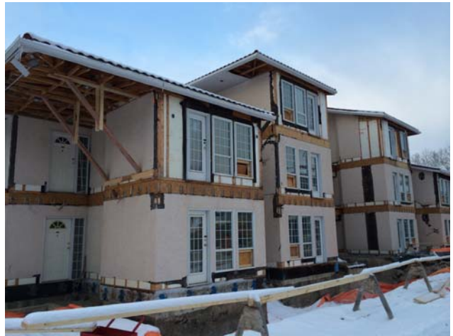
Views of the north (front) elevation of Building 300. Exterior demolition work is generally complete.
