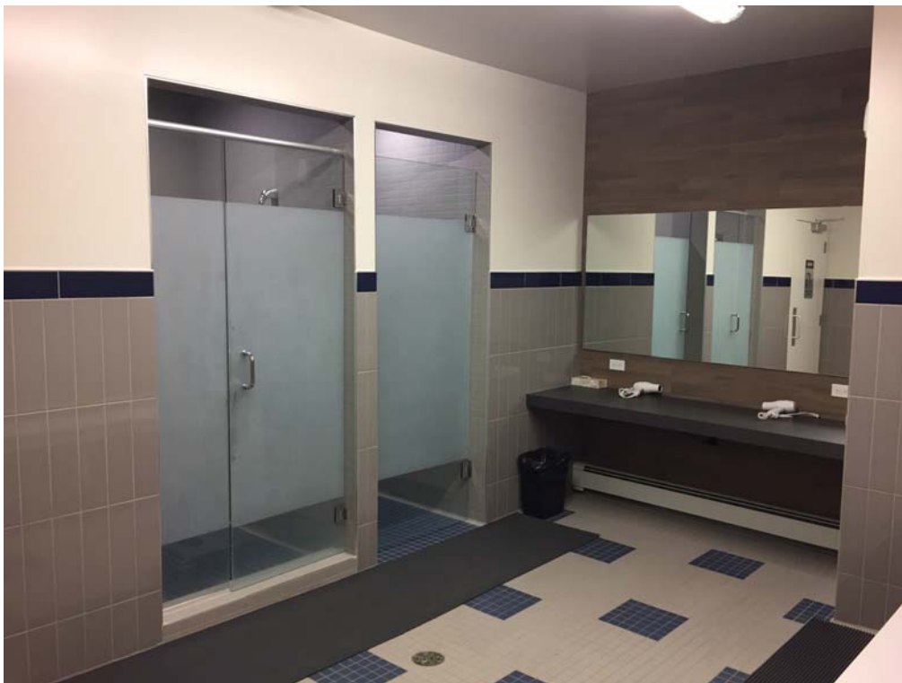
The ladies change room shower glass doors and mirrors have been installed.
