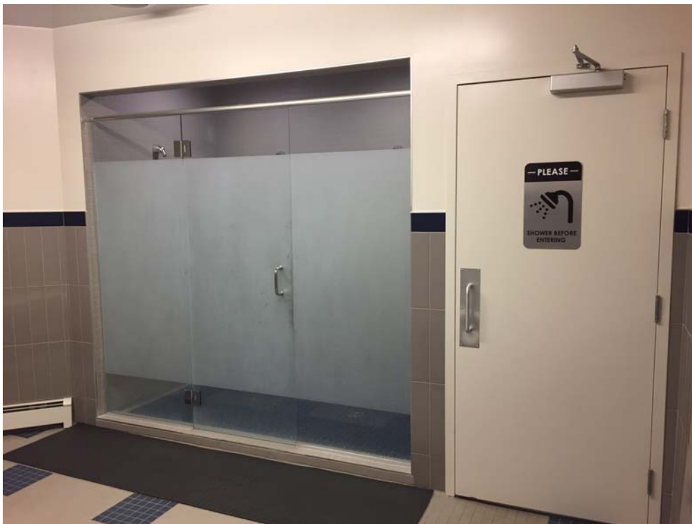
The men's change room shower glass door and partitions have been installed.
