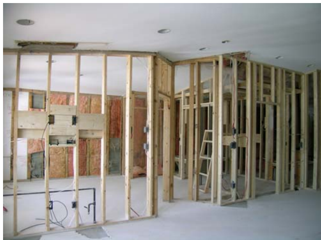
Building 400 – All of the framing has been completed. Insulating is well advanced.
