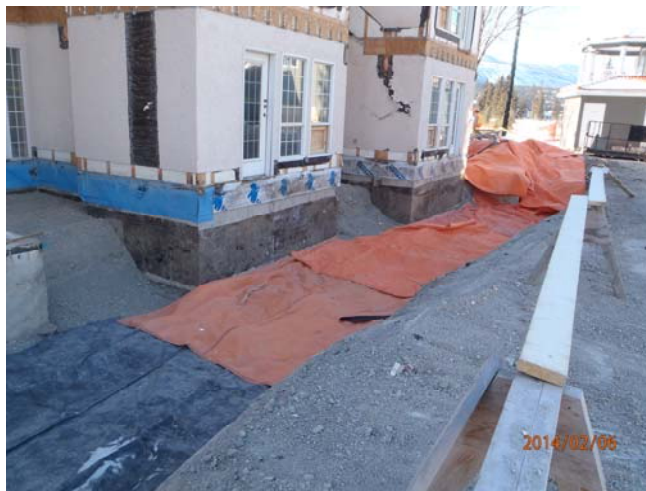
Building 300 Exterior Slab re-construction.
