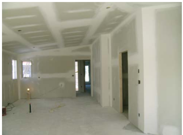
Building 300 – Doors and frames have been delivered. Drywall finishing work is nearly complete.
