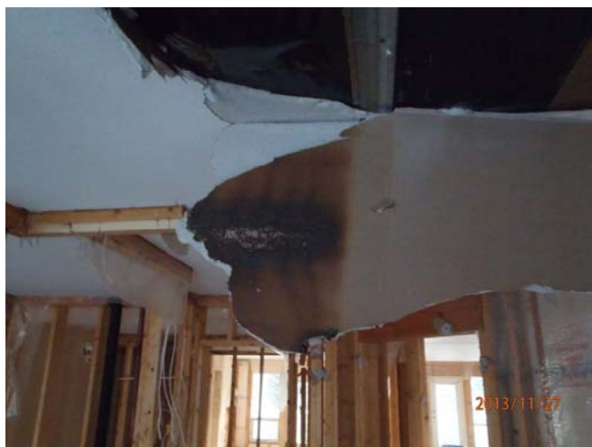
Building 300 failed former electrical heating system.
