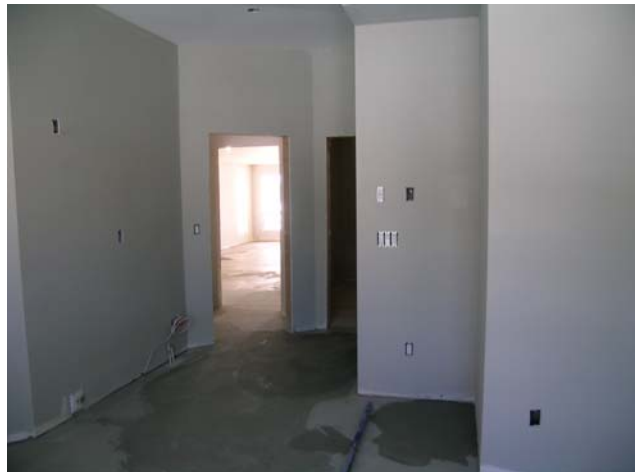
Building 300 – Rough-in work is complete. Finish painting is well advanced.
