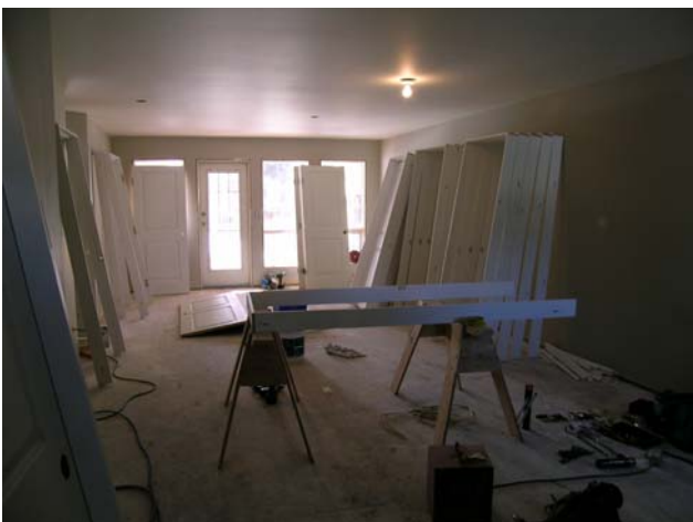
Building 300 – Doors and frames have been delivered. Drywall finishing work is nearly complete.
