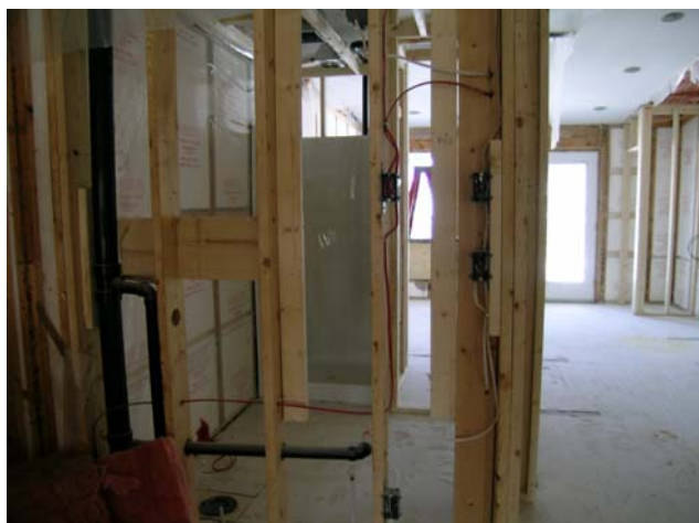
Building 400 – The new plumbing rough-in is well underway.
