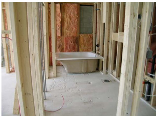
Building 400 – The new tubs are on site. Electrical rough-in work is generally complete.
