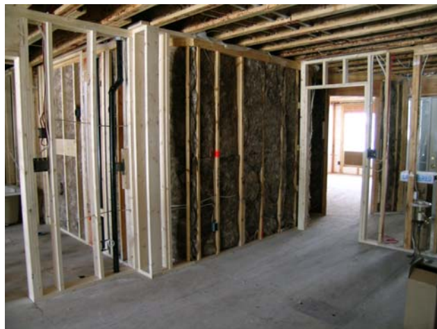
Building 400 – All of the framing has been completed. Insulating is well advanced.
