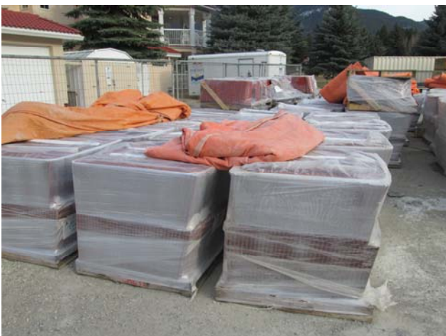
The new building 300 roof tiles have been delivered.
