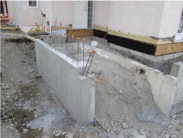
Views of the new concrete grade beams and foundation walls along the north side of building 300.
