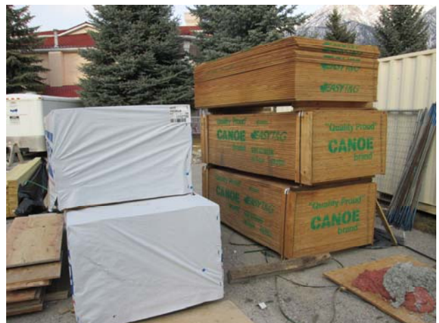
View of the additional framing materials on site.
