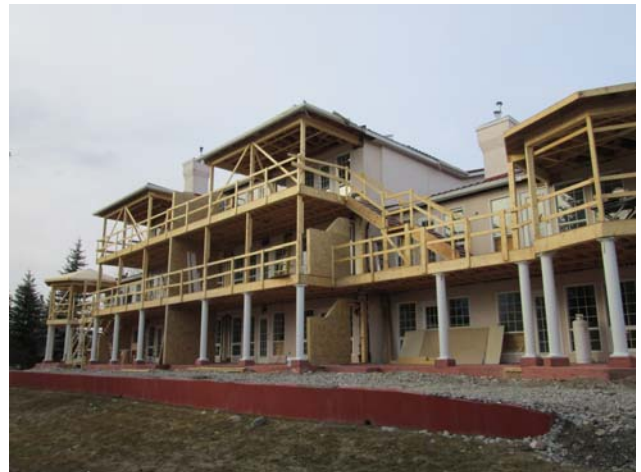
Views of the south elevation of building 300. Framing of the new balconies is generally complete.
