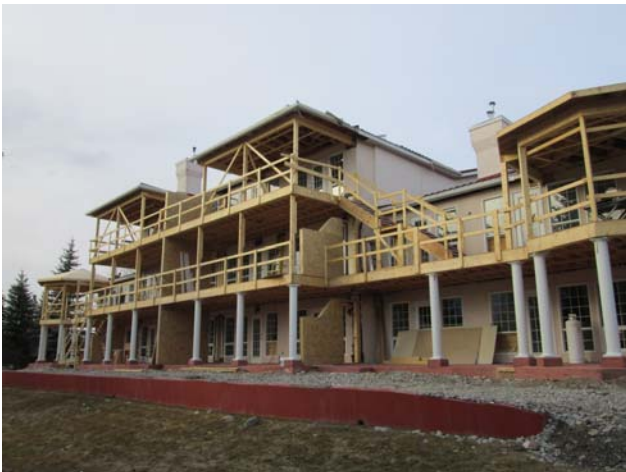
Views of the south elevation of building 300. Framing of the new balconies is generally complete.
