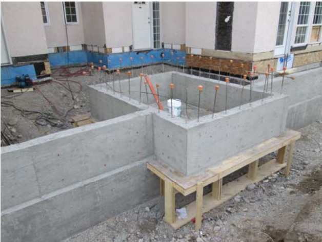
View of the new central stair foundation walls.
