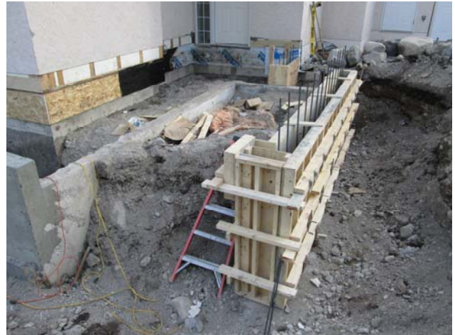
One section of foundation wall remains to be poured.
