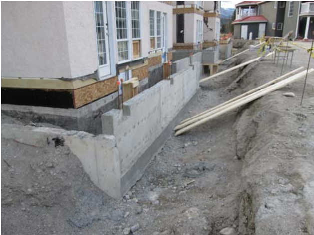
Views of the new concrete grade beams and foundation walls along the north side of building 300.
