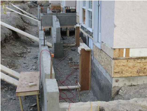
Further view of the new foundations.
