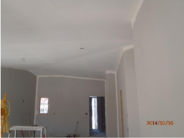
Building 300 – Typical Interior: All plumbing and electrical components removed and replaced. Units re-dry walled and awaiting paint.
