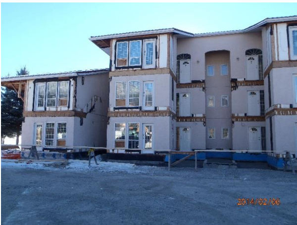
Building 300 Exterior Work – Patios, Decks and Stairs Removed
