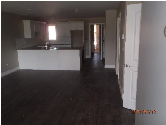
Building 400 – Interior Progress: A and B Sides
