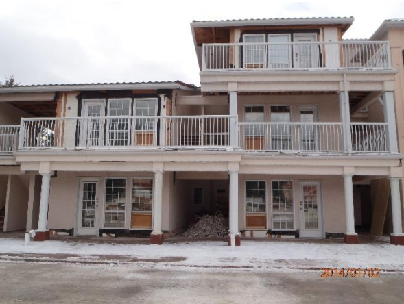
Building 300 Exterior Work – Removal of Stucco in Preparation for Deck and Patio Removal
