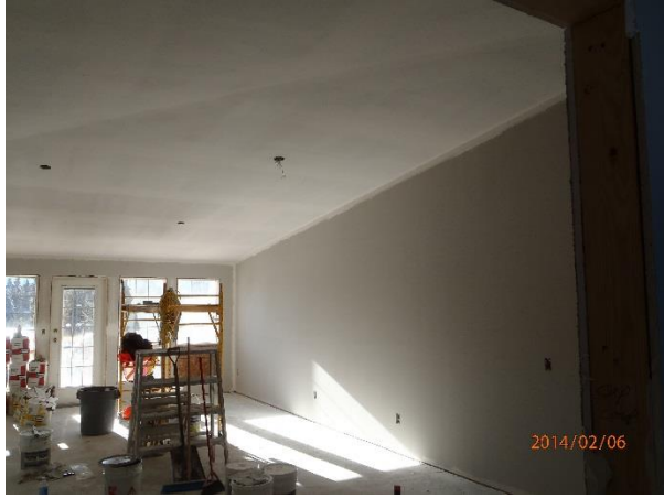
Building 300 – Typical Interior: All plumbing and electrical components removed and replaced. Units re-dry walled and awaiting paint.
