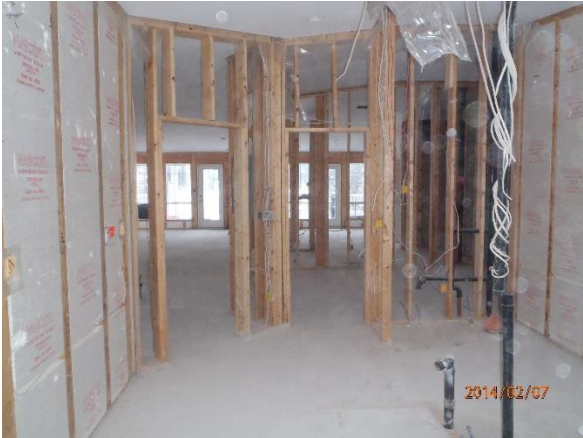
Building 400 – Interior Demolition
