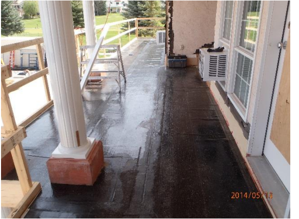
Building 300 – New Deck and Membrane Application
