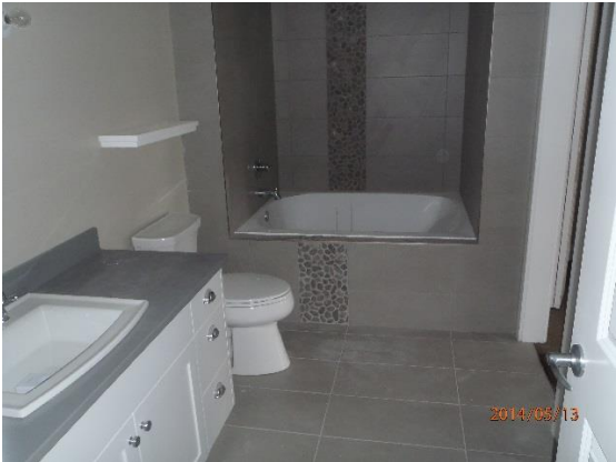
Building 400 – Interior Progress: A and B Sides
