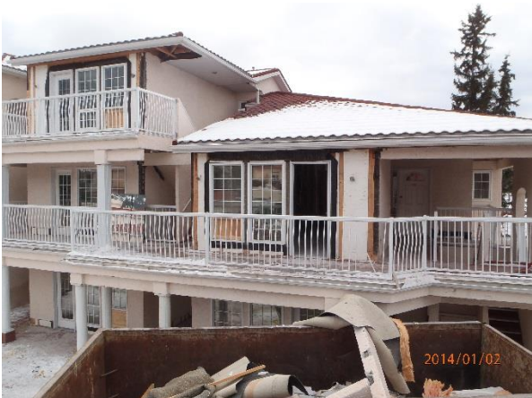
Building 300 Exterior Work – Removal of Stucco in Preparation for Deck and Patio Removal
