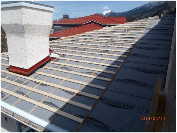
Building 300 – New Roof Installation and New Deck Construction
