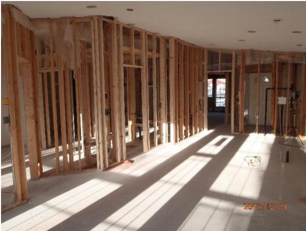
Building 300 – Interior Demolition and Removal of Poly B Plumbing and Electrical Service
