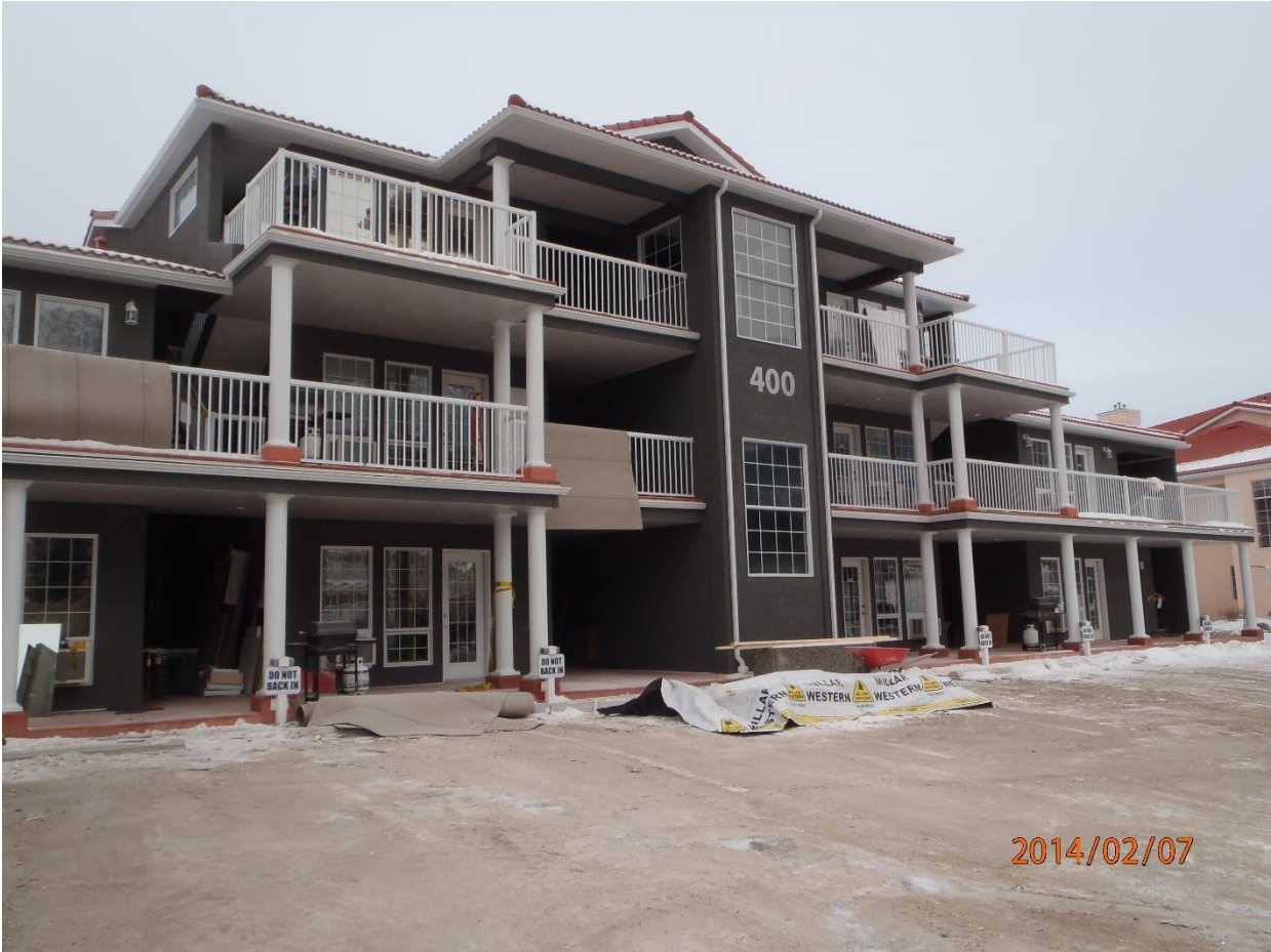
Building 400 – Exterior Complete
