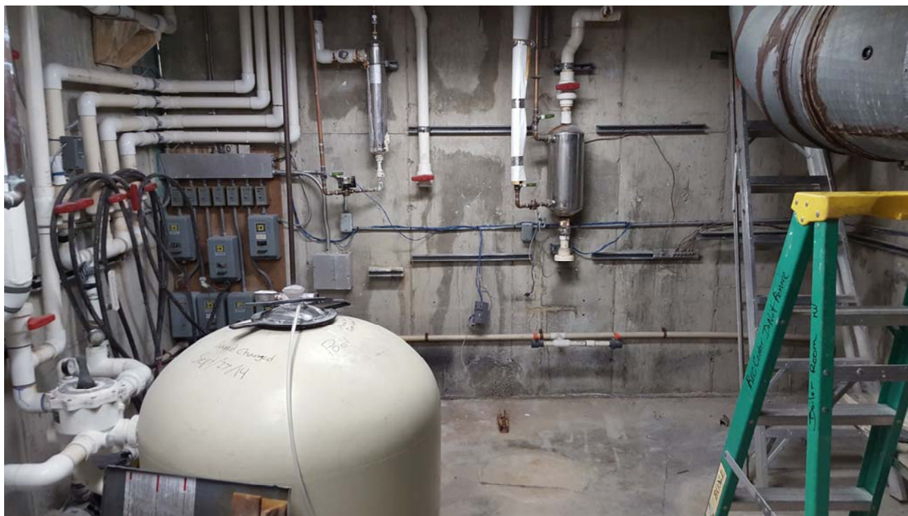
View of the basement mechanical room. The existing pool equipment has been removed.
