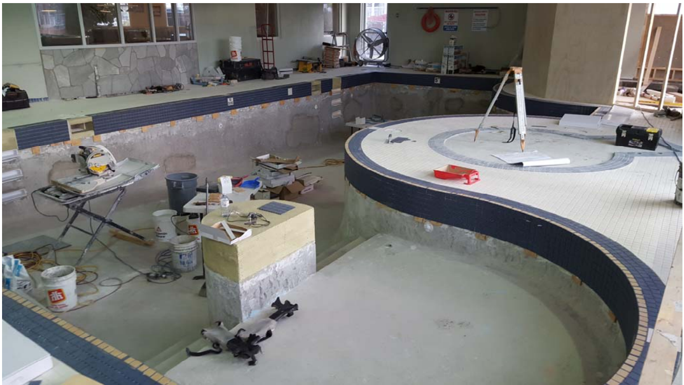
View of the existing indoor swimming pool. The existing pool tile has been removed.
