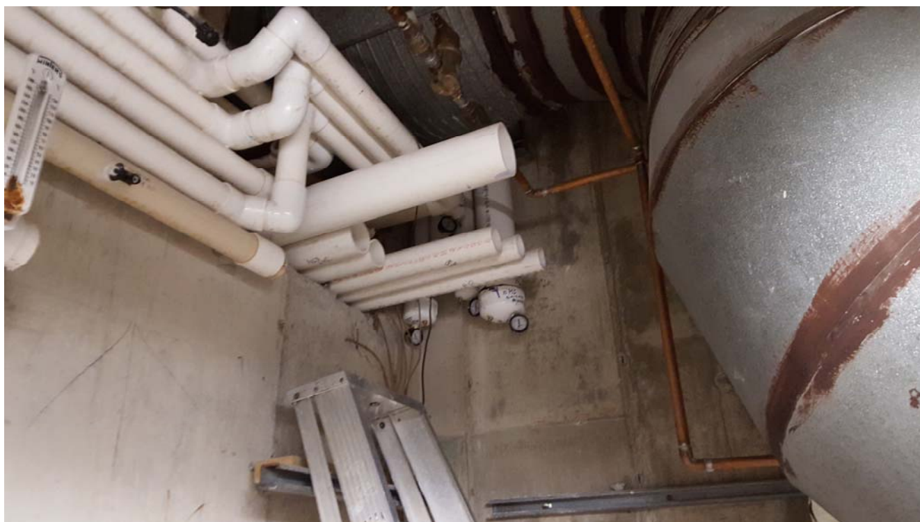
View of the new plumbing routed to the mechanical room from the new whirlpools.
