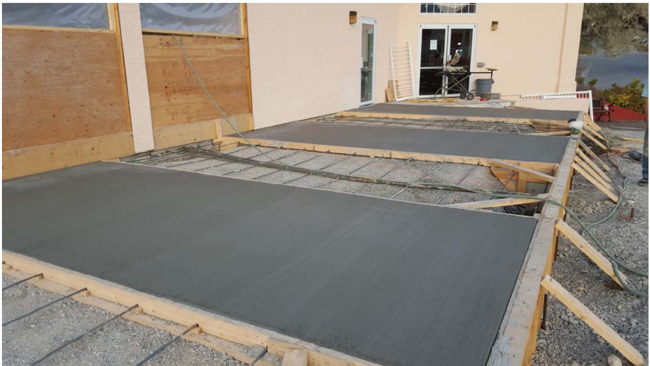
Placing of the new concrete patio is well advanced on the south side of the building.
