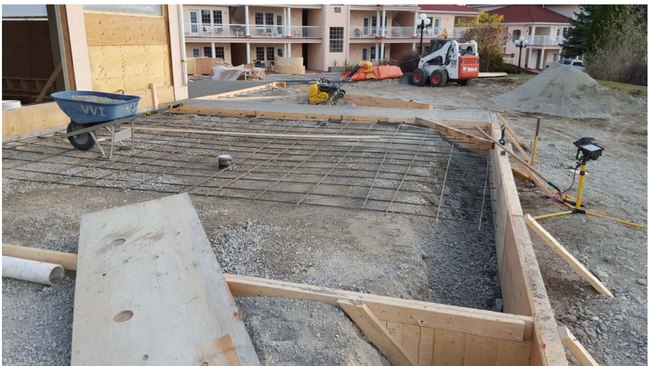
View of the patio area on the west side of the building. Placing of the concrete slab rebar is underway.
