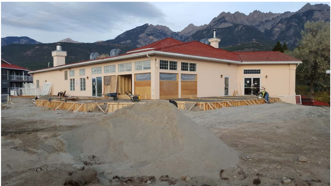
The existing concrete sidewalk, patio, and stairs have been removed
