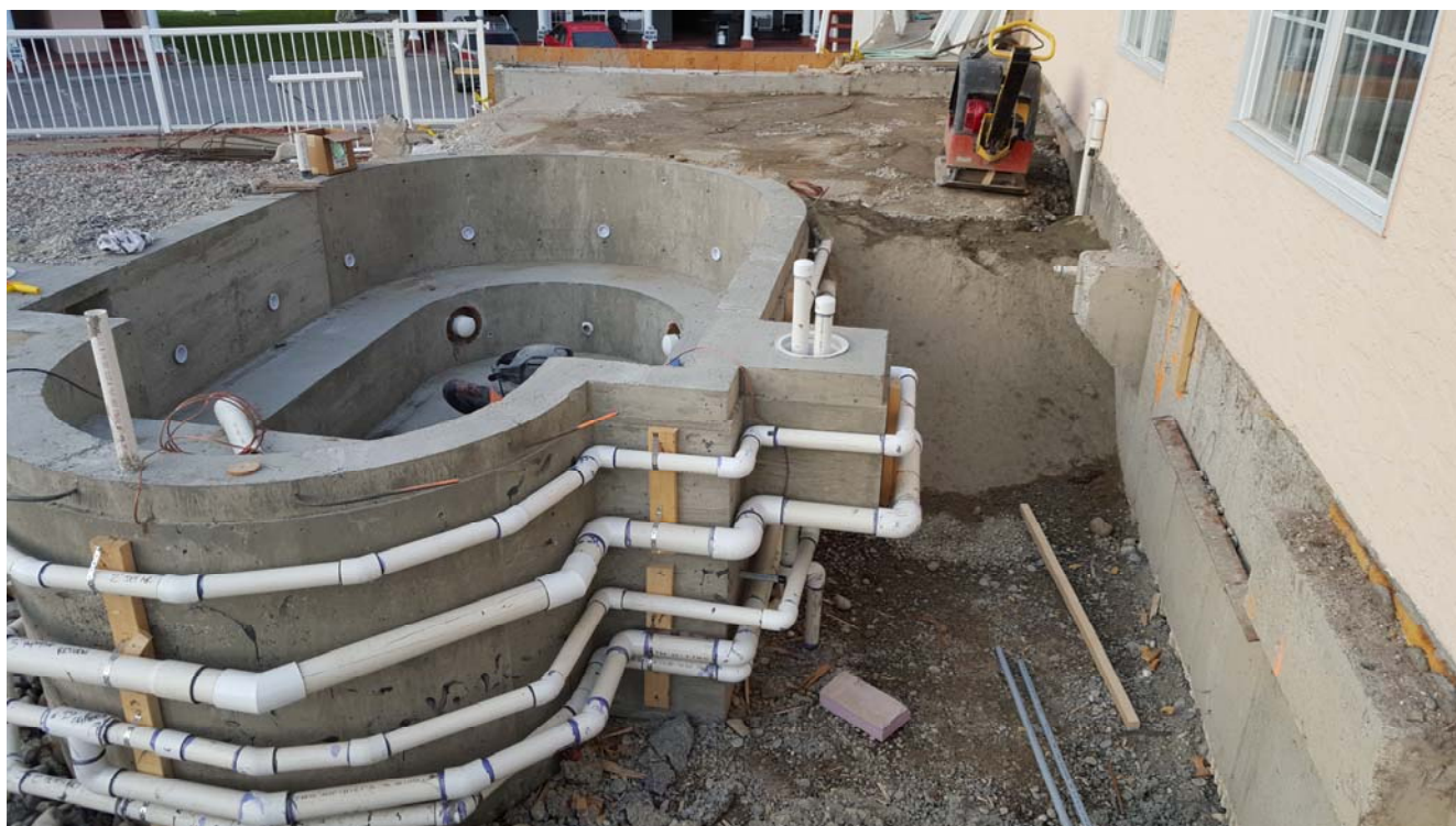
The new exterior whirlpool has been cast, the plumbing has been installed, and backfilling is underway.
