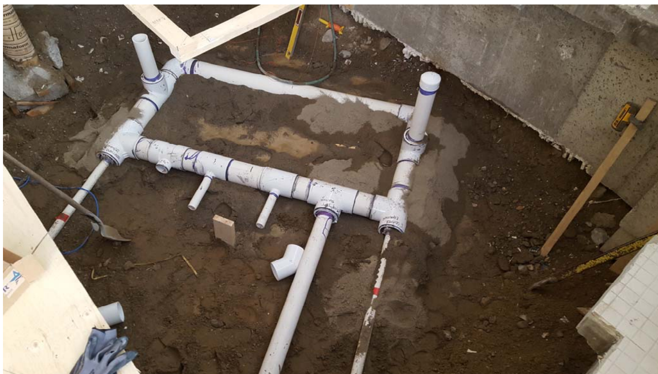
Installation of the new supply and return plumbing for the new whirlpool is nearly complete.
