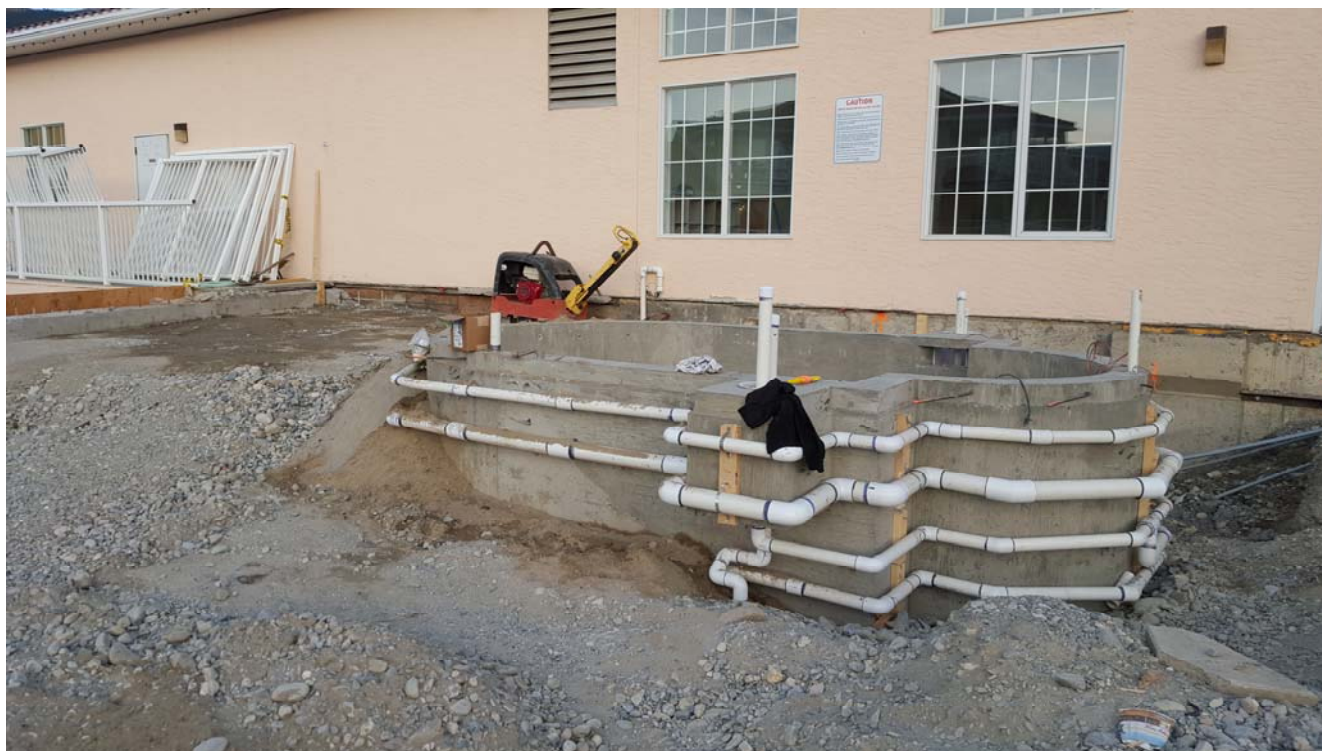
View of the new exterior whirlpool on the west side of the building.
