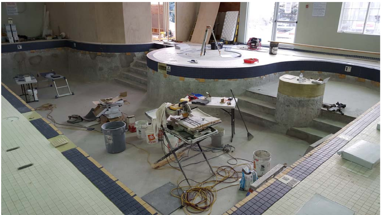
The new trim tile and markers have been placed around the perimeter of the pool (grouting to be completed).
