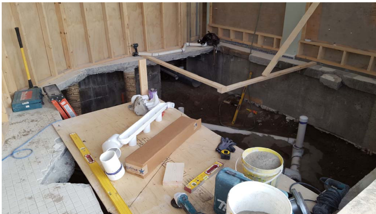
The existing suspended concrete slab has been removed for the installation of the new whirlpool.
